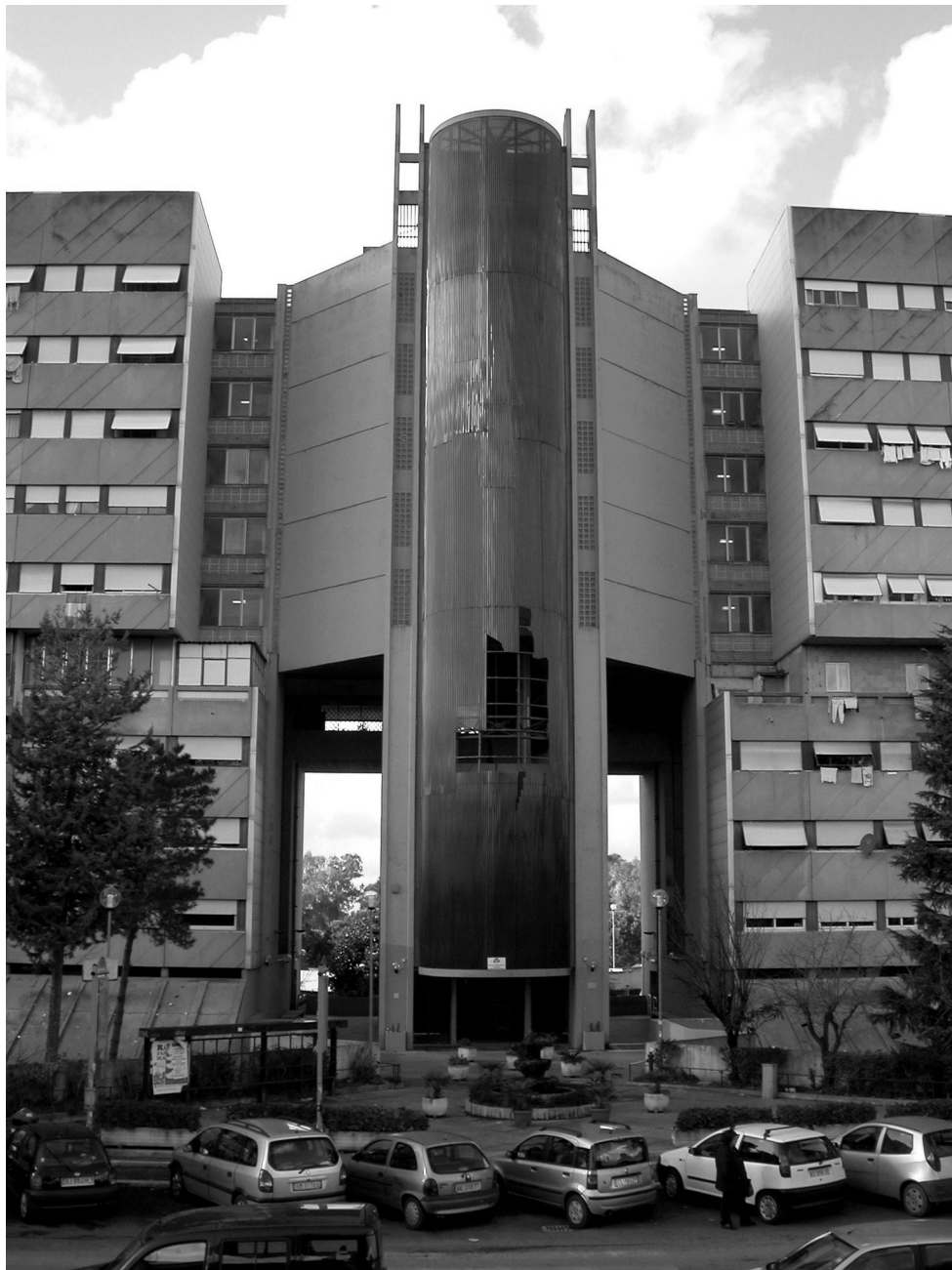
Fig. 3 The elevators frequently malfunctioned and, along with the entryways, were often targeted by vandals. By late 1983, nearly 700 families were illegally occupying the building. The squatters settled into the fourth floor of the main building, which had originally been designed to support boutiques for artisan products, offices and commercial activities. This design strategy emulated the modern housing typology of the Unité d'Habitation, designed by Le Corbusier in the early 1950s.
