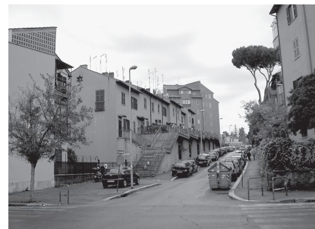
Fig. 1 Tiburtino Housing Project, Rome (1949-54) Project Architects: Ludovico Quaroni, Mario Ridolfi (lead architects); Mario Fiorentino, Federico Gorio, Maurizio Lanza, Piero Maria Lugli, Giulio Rinaldi, Michele Valori with Carlo Aymonino, Carlo Chiarini, Sergio Lenzi, Carlo Melograni, Gian Carlo Menichetti. Many of the architects who worked on the Tiburtino project were members of the Rome-based Association for Organic Architecture (APAO).
