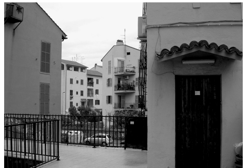
Fig. 4 The casual front entrances along the raised walkway were intended to produce more intimate thresholds between public, semi-public, and private domestic spaces. The scale and detailing of the door stoops and awnings mimic the vernacular character and ambience of an Italian village. It was imagined that the design would better suit the future inhabitants of the state-sponsored housing project.
