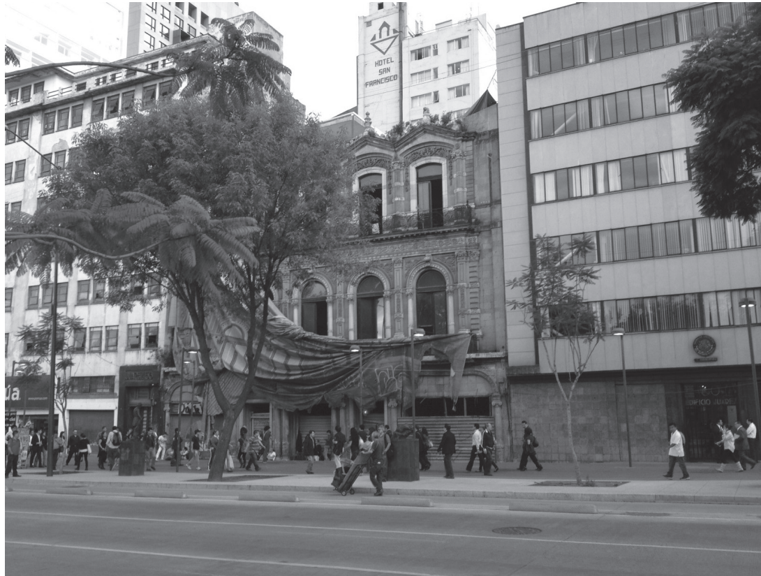
Abandoned historic building, Avenida Juárez
