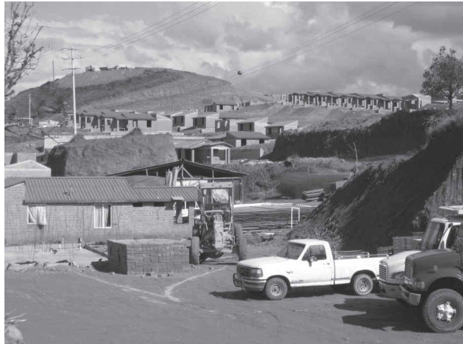
Sustainable Rural City Nuevo Juan Grijalva, Chiapas, being built.
