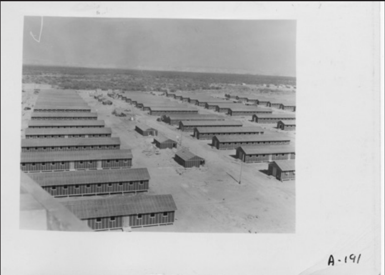
Figure 63: Block units of fourteen barracks and communal mess halls, laundries, and latrines built to Army standard specifications, June 1, 1942. Courtesy of The Bancroft Library
