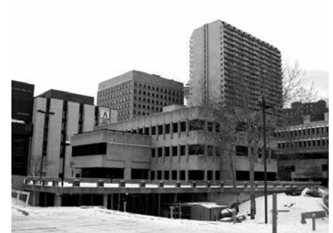
Figure 6. Several blocks were converted to massive institutional buildings (shown here the Board of Education Building, with the Public Library in the left background, on Macleod Trail and 5th Avenue SW) that do not positively contribute to the public realm. Photo F. Shaw 2005.
