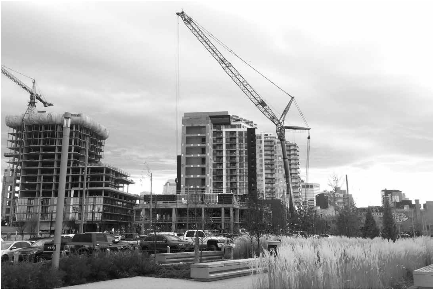
Figure 8. The public realm and river path were constructed in advance of the residential development in the East Village. Photo B. Sandalack 2017.
